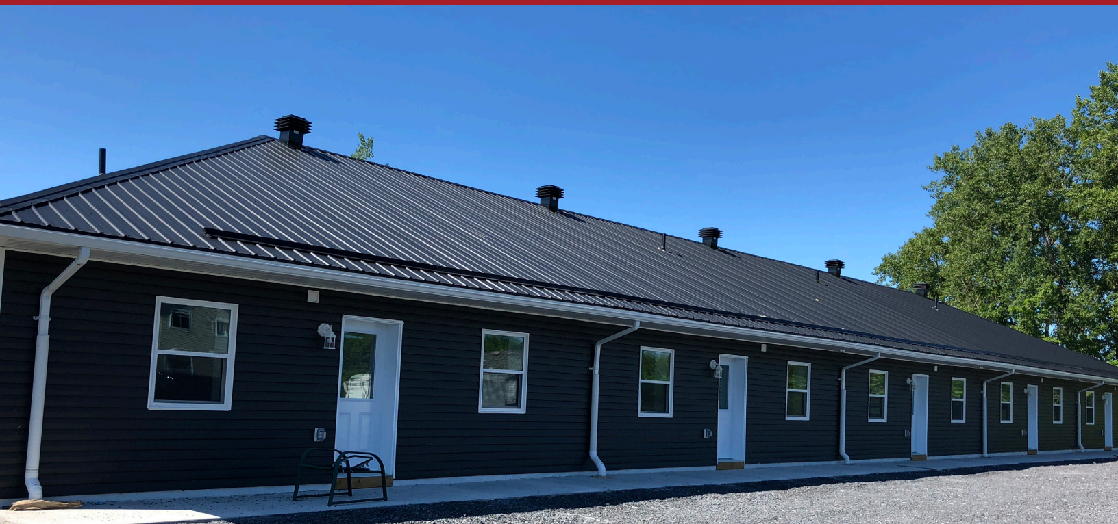
Energy efficient five plex built in by the Mohawk Council of Akwesasne. Photo by Corey Tarbell.
